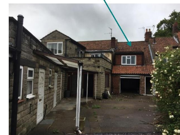
Image 3 View from 'yard area' looking towards Eastgate showing rear of Greystones
