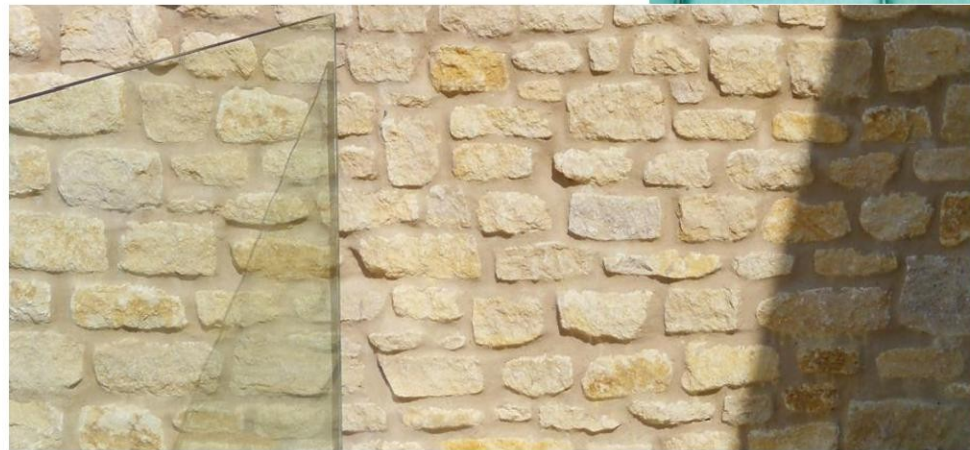
Random rubble stone to Courtyard level of Multi-Use Rooms/Coffee Yard
